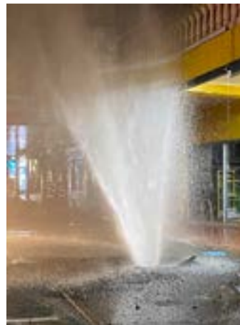
Burst water main on Pollen St.
