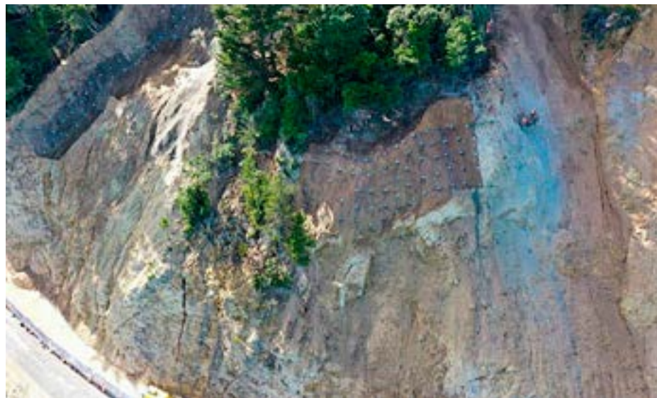
Workers clear debris and install soil nails and mesh on the cliff face. Photo: SUPPLIED
