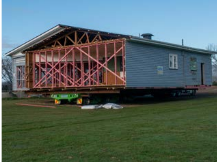
The first half of the building in its new location, left. The second half at the old location, in preparation to be loaded on to the moving truck.
