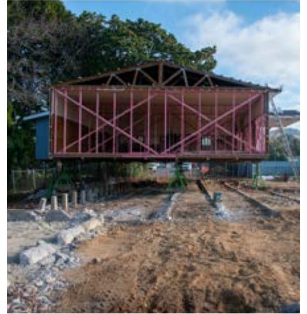
The first half of the building in its new location, left. The second half at the old location, in preparation to be loaded on to the moving truck.
