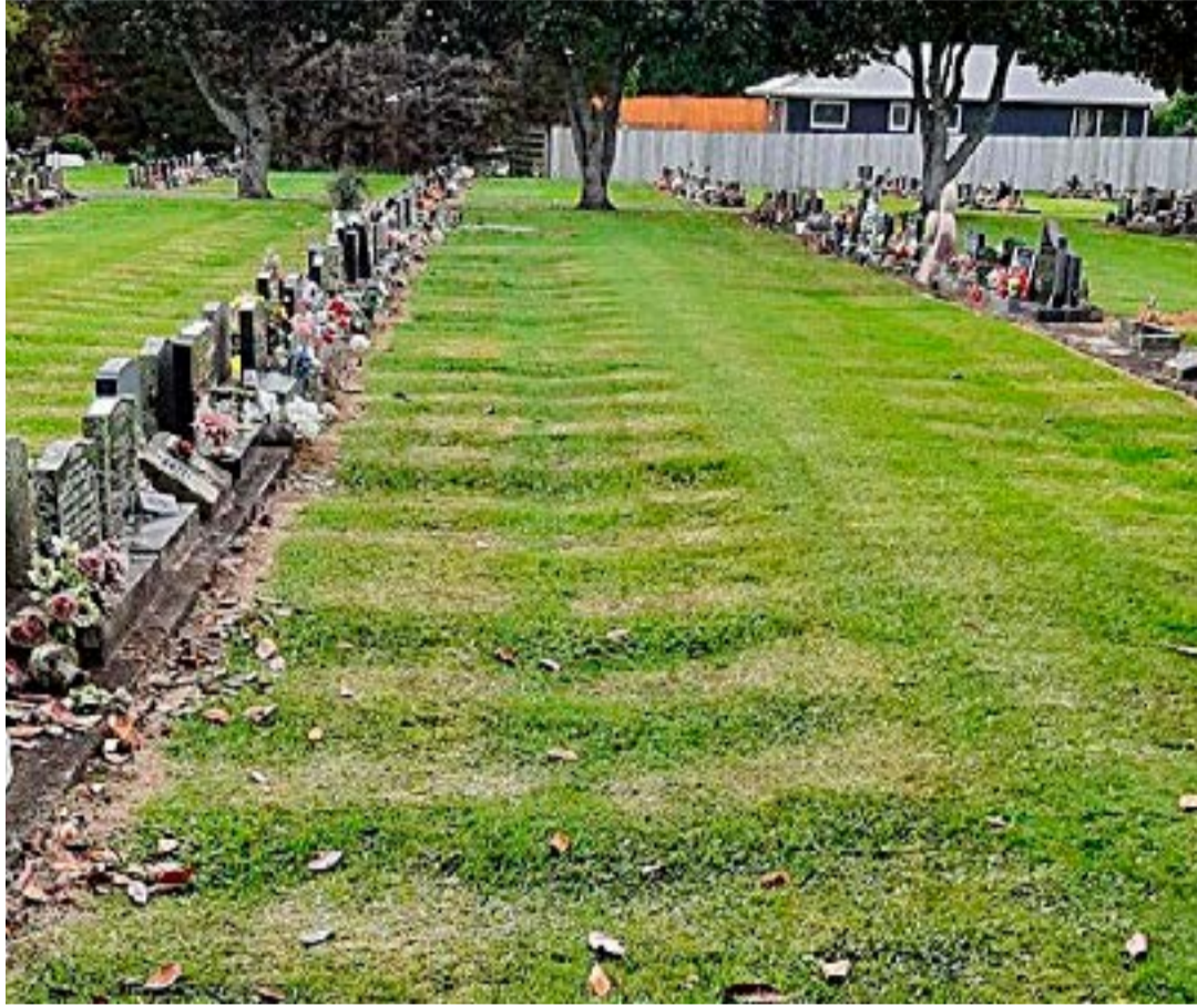
Subsidence at Waihi Cemetery.
