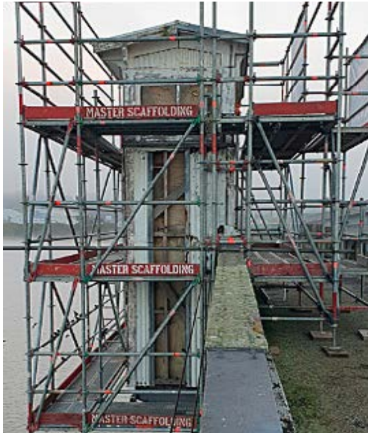
The Historic Kōpū Bridge wheelhouse before and after recent restorations.
