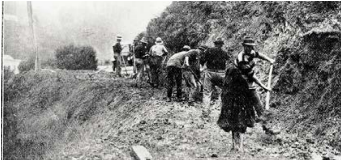
Clearing a slip on the Waihi Road at Karangahake.
