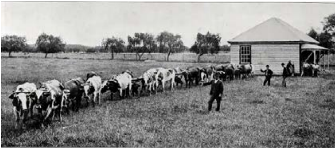
On the move at Hikutaia - shifting a six-roomed house by bullock team.
