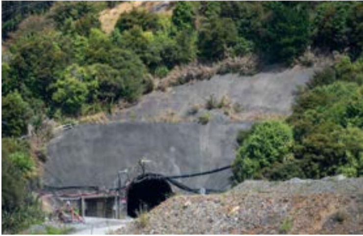
The underground mine portal, heading into the underground mine.
