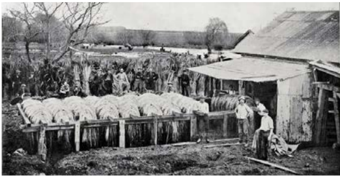
Flax fibre on skids at Kerepēhi ready for the drying paddock.
