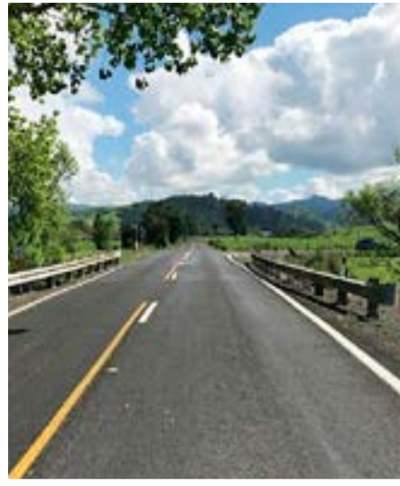
The Onetai Stream Bridge along SH26, north of Paeroa, is getting replaced.
